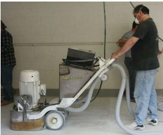
Grinder with local exhaust attachment
